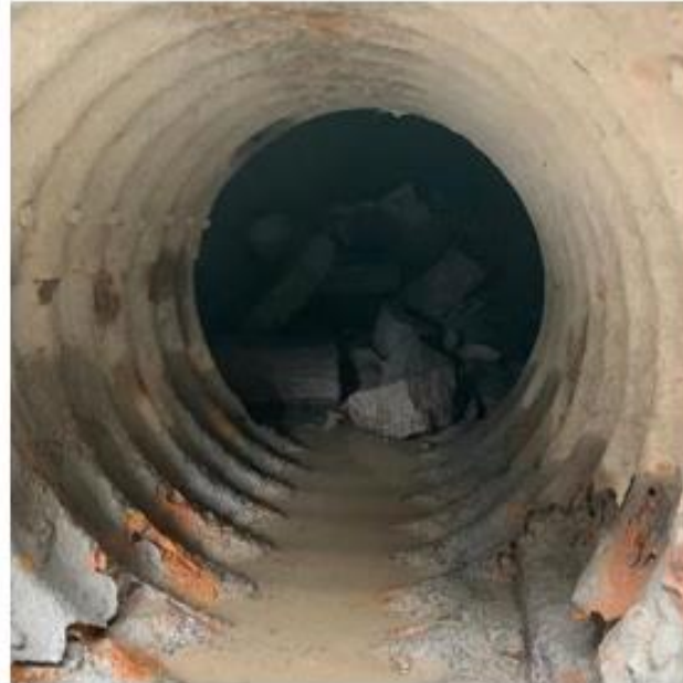
Fig 6 Woodlands tidal outfall on Thurs 2 Sept 2021 – left photo headwall now disintegrating and right photo blocked cul
