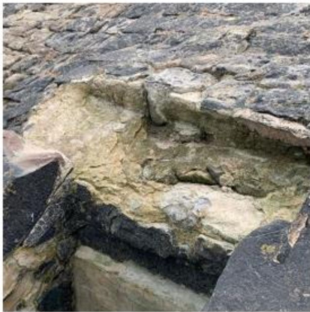
Fig 6 Woodlands tidal outfall on Thurs 2 Sept 2021 – left photo headwall now disintegrating and right photo blocked cul
