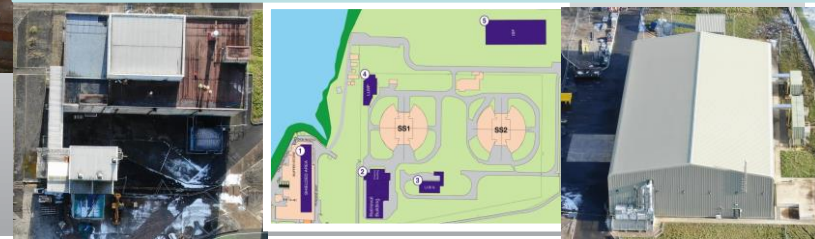
Other Building Demolition
