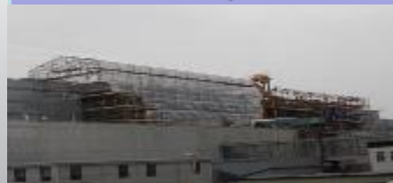
Non RCA South Clearance (inc. Turbine Hall)
