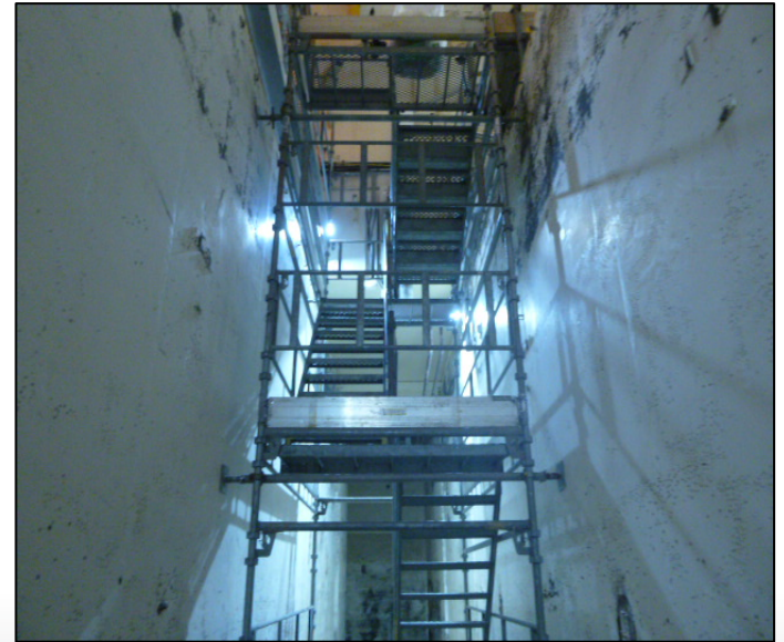
“Haki” staircase installed to enable easier access
