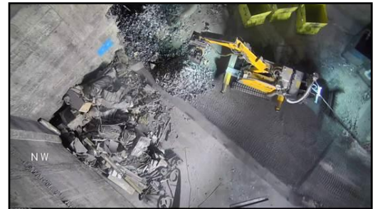
Bunker Waste Recovery Operations, showing a Brokk sorting waste from Bunker 1
