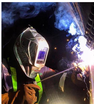
Mona Group undertaking pipeline
