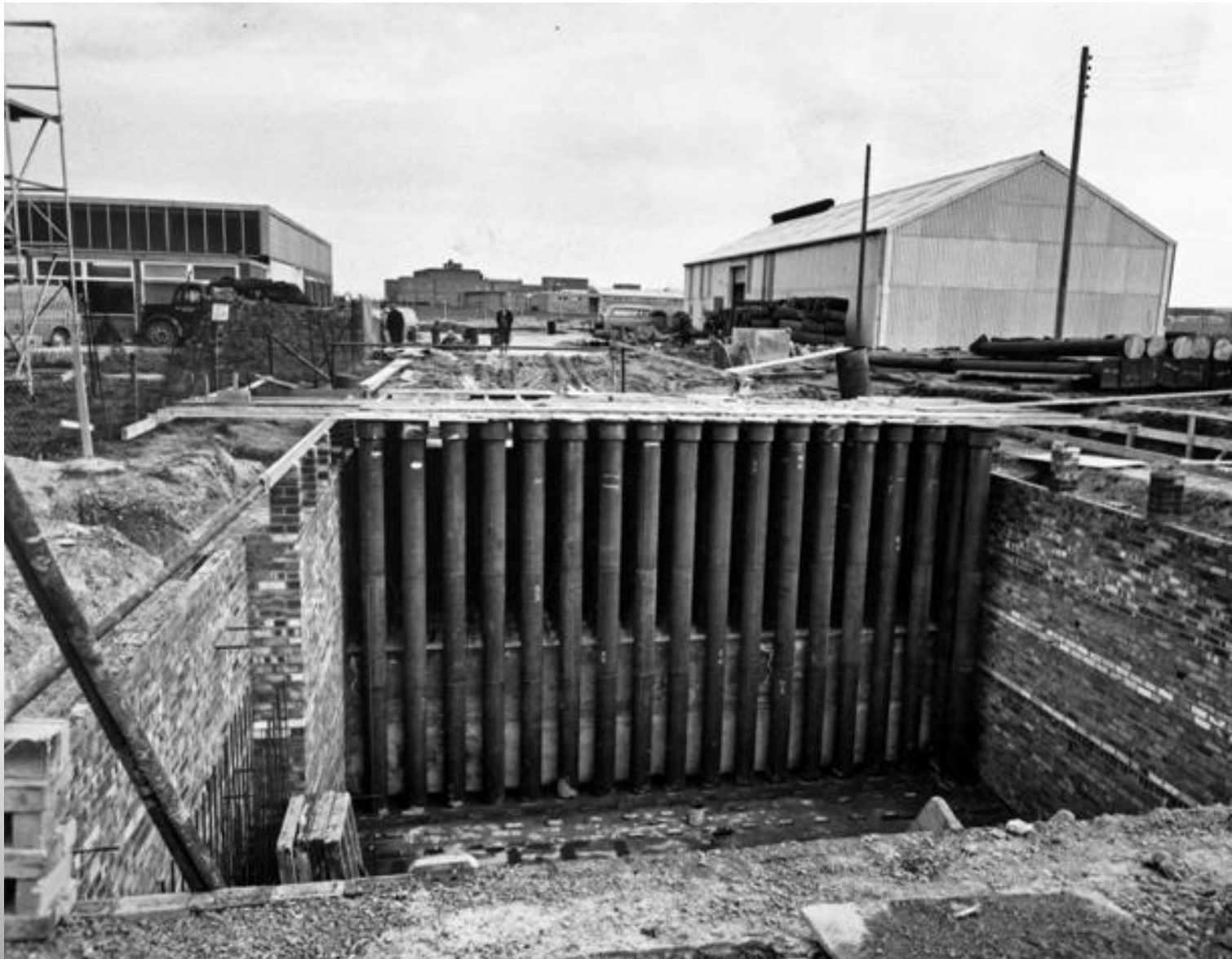
Tube Store during construction
