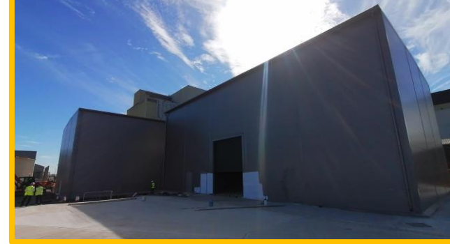
Wet Waste Bldg (B134)
