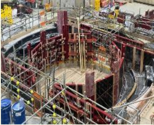
Formwork installed & concrete poured 169' Overcore
