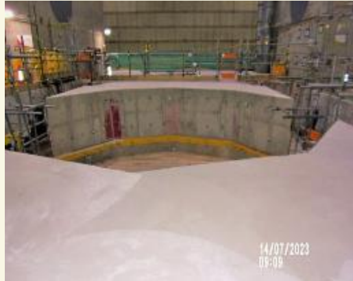
Formwork installed & concrete poured 169' Overcore
