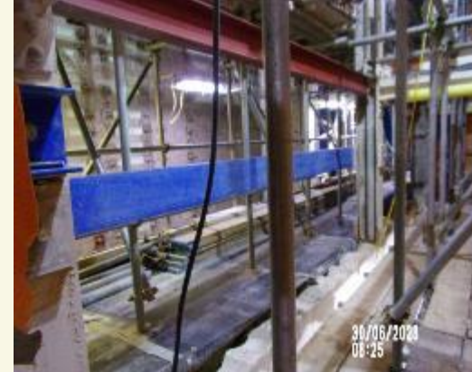
Robot access penetration cut North Annexe
