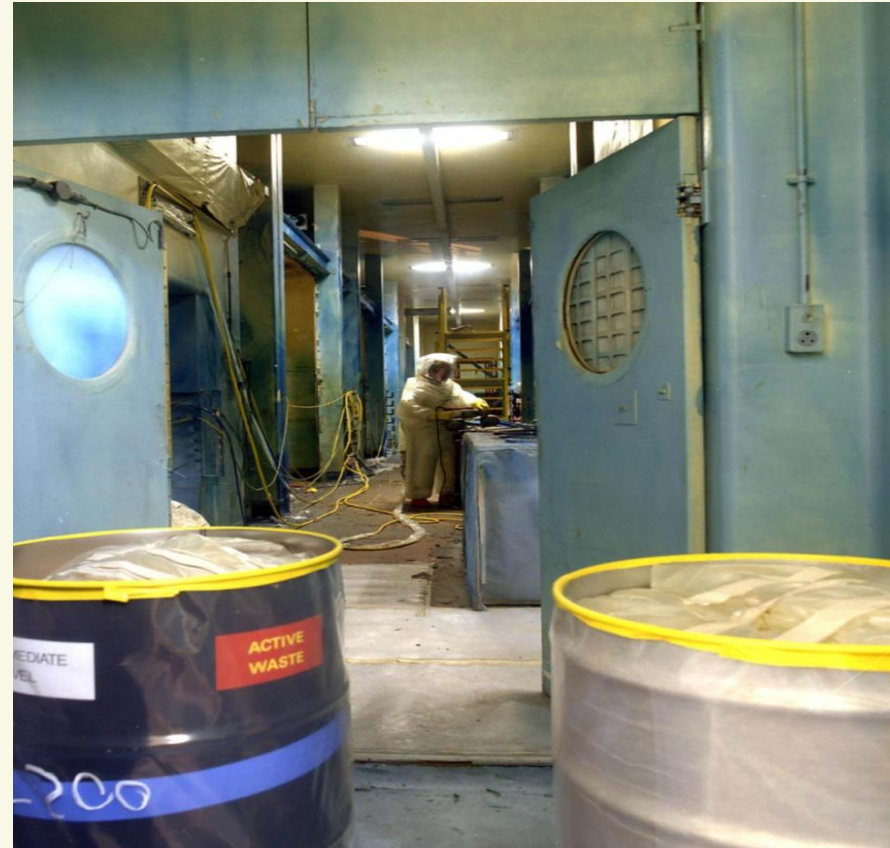
Pressurised suit work
