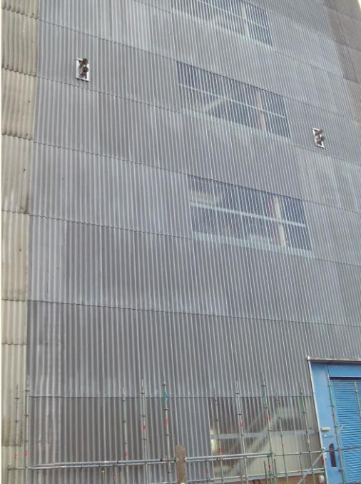
Reactor 1 South Face Complete
