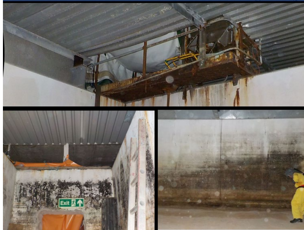
Internal views of Delay tanks
