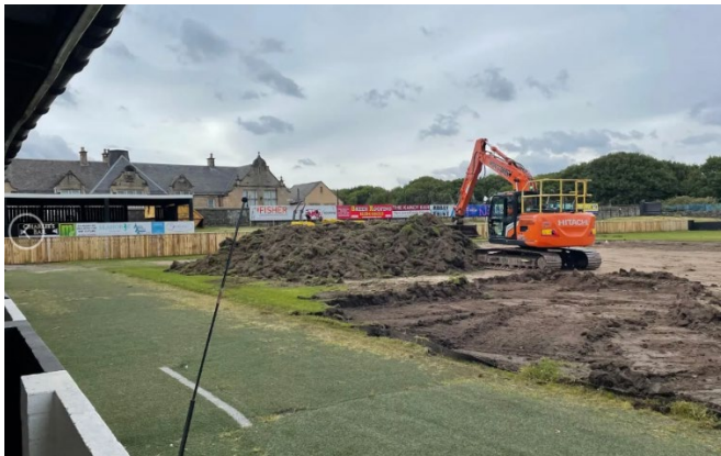
Work commenced replacing the pitch
