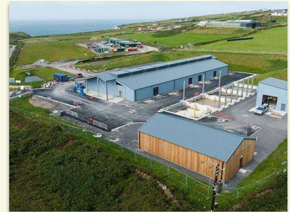
Sub-station at South Stack officially opened by The First Minister of Wales Mark Drakeford in October 2023
