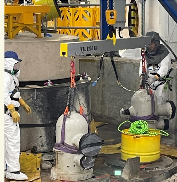
Removal of shielding from coolant ducts
