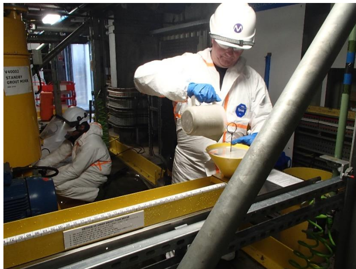
Grouting trials underway
