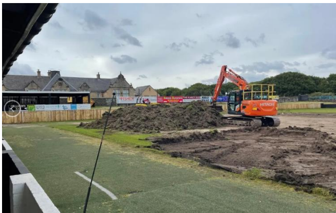
Work commenced replacing the pitch
