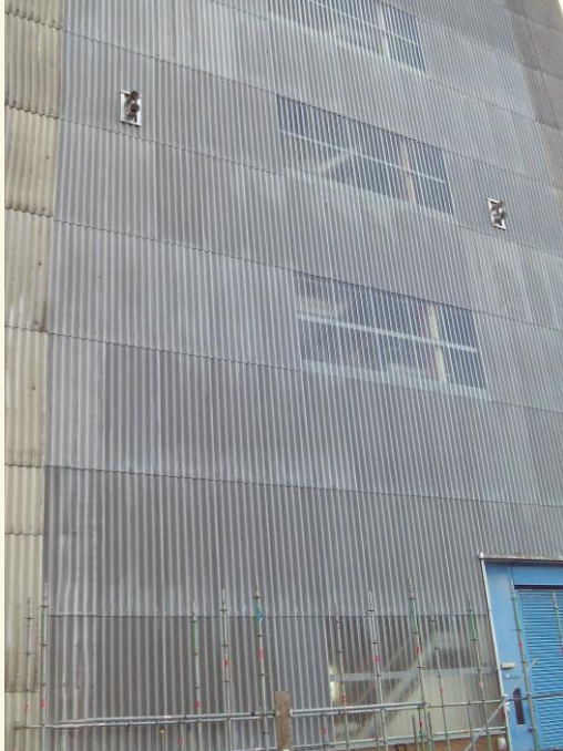
Reactor 1 South Face Complete
