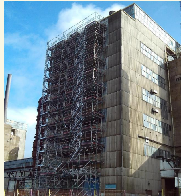
Reactor 3 – Scaffolding Complete
