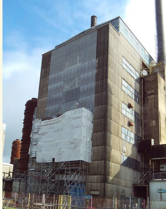
Reactor 2 – Glazing Replacement in Progress
