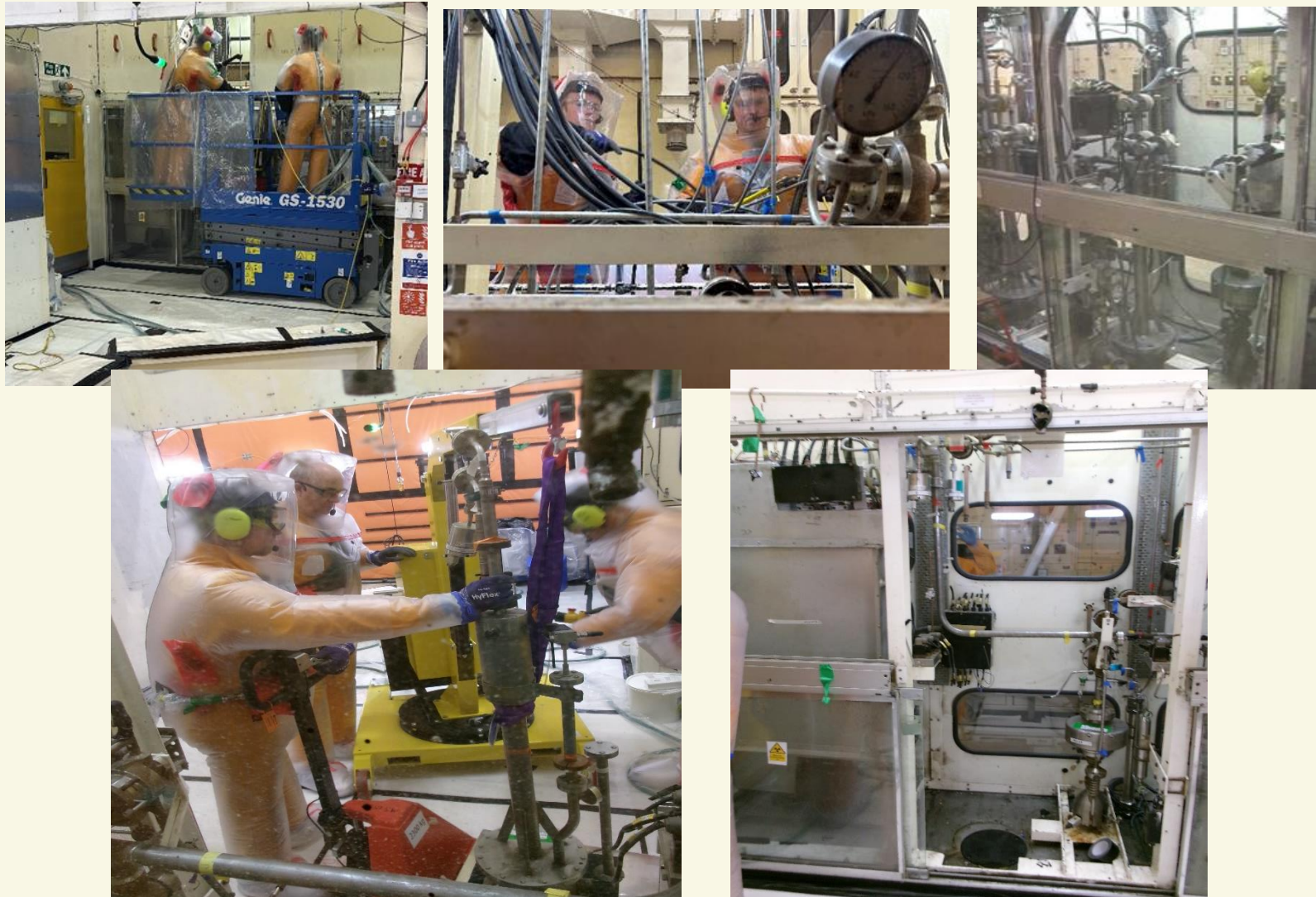
Cleaning, soft strip and de-planting operations as part of Process Line Active commissioning
