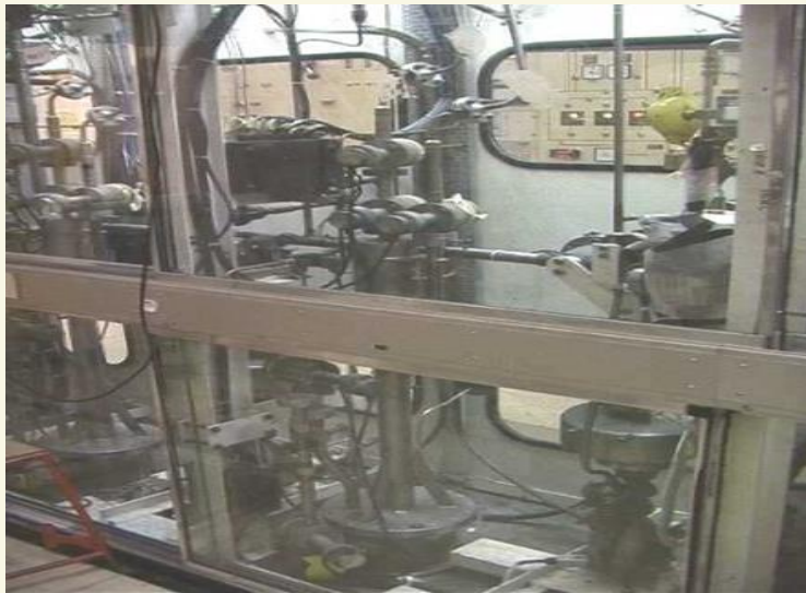
Contaminated Tritium Purification Vessels and Pumping Systems Within the Process Cubicle
