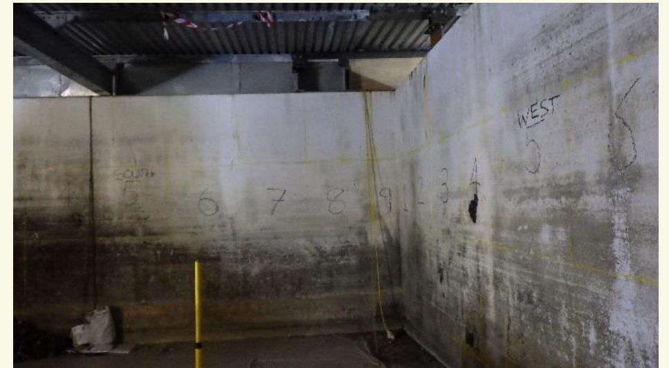
Divide wall between delay tanks 1 and 2 with the temporary scaffold supports now removed
