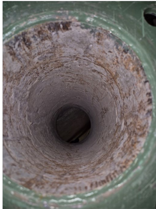
After - powder delivery pipe clear
