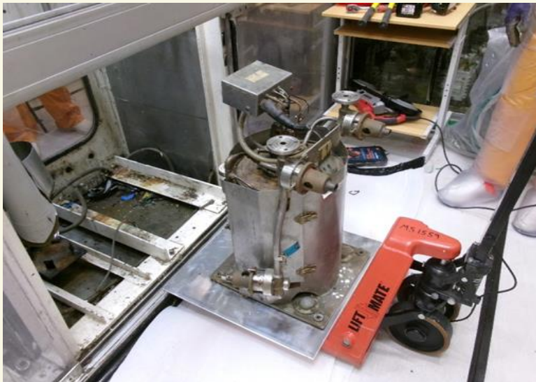
Retrieval of tritium contaminated Uranium Furnace from Process Cubicle and size reduction
