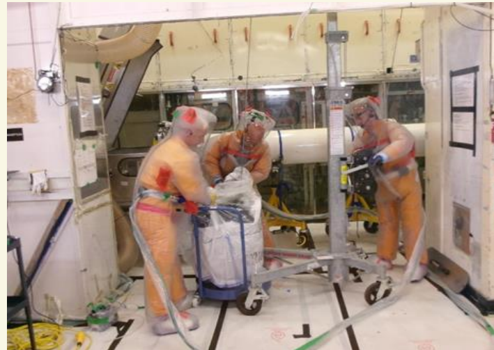
Removal of cut section from Cutting Box and packaging into a FIBC
