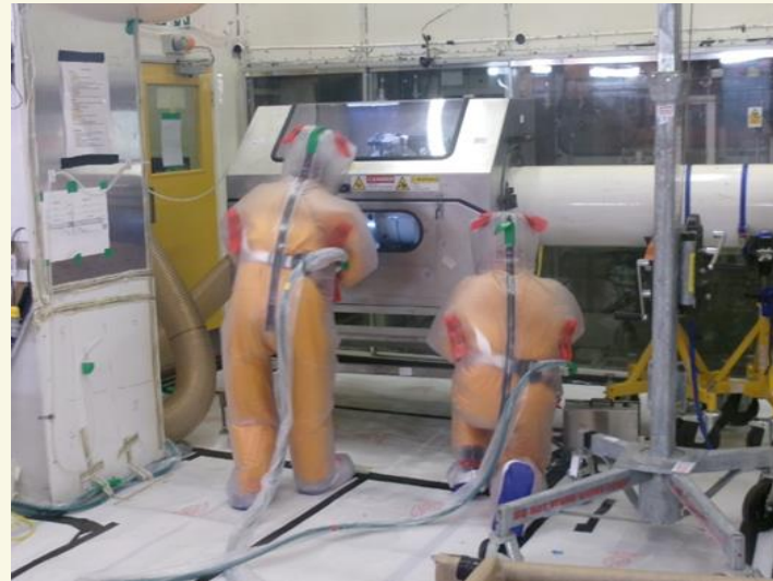
Setting up Orbital Cutter within the Ventilated Cutting Box to size reduce the VPE Tank
