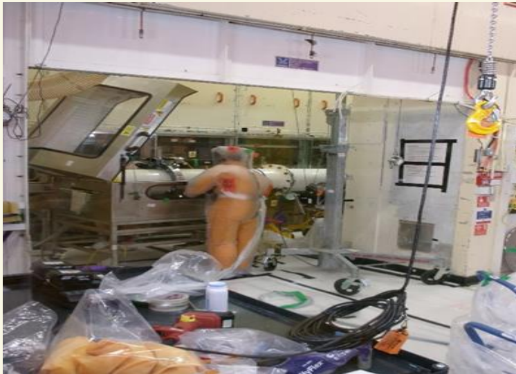
Setting up Orbital Cutter within the Ventilated Cutting Box to size reduce the VPE Tank
