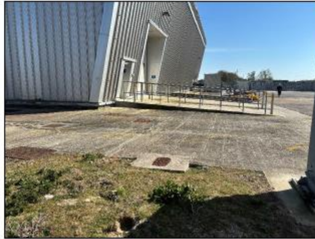
Figure 2, Ramp to the raised ISF floor
