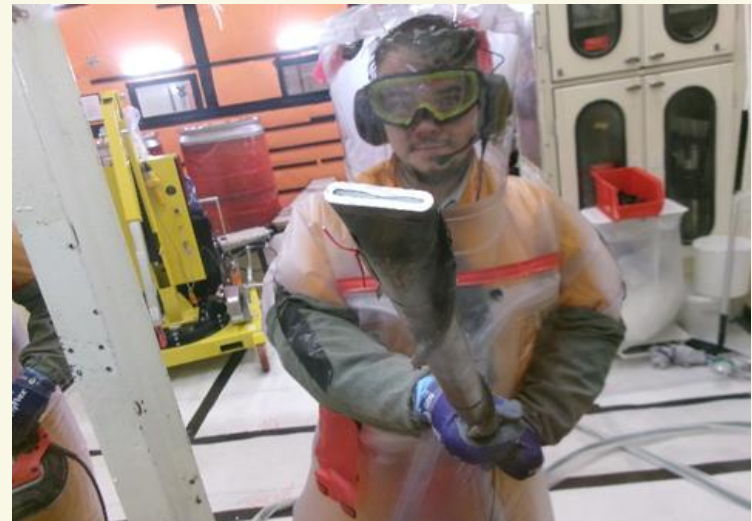
‘Crimp & Cut’ methods used to reduce tritium discharge and retain column packing materials
