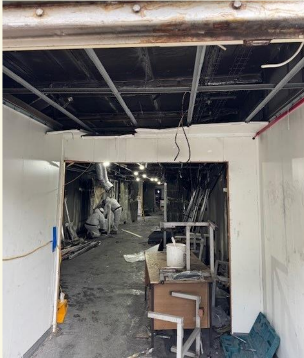
Change facility strip out in progress
