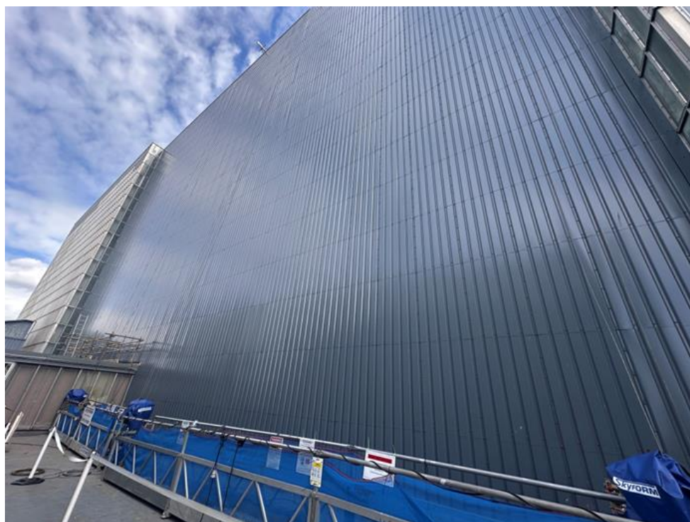
Charge Hall North Side Elevation
